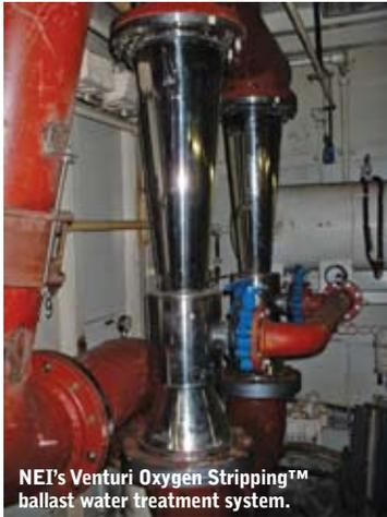
NEI's Venturi Oxygen Stripping™ ballast water treatment system.
